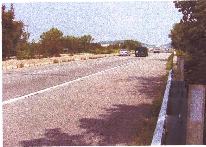
ACROSS TOP, OF DECK
