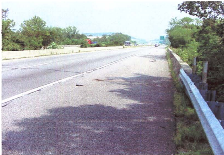
Across Top of Deck
