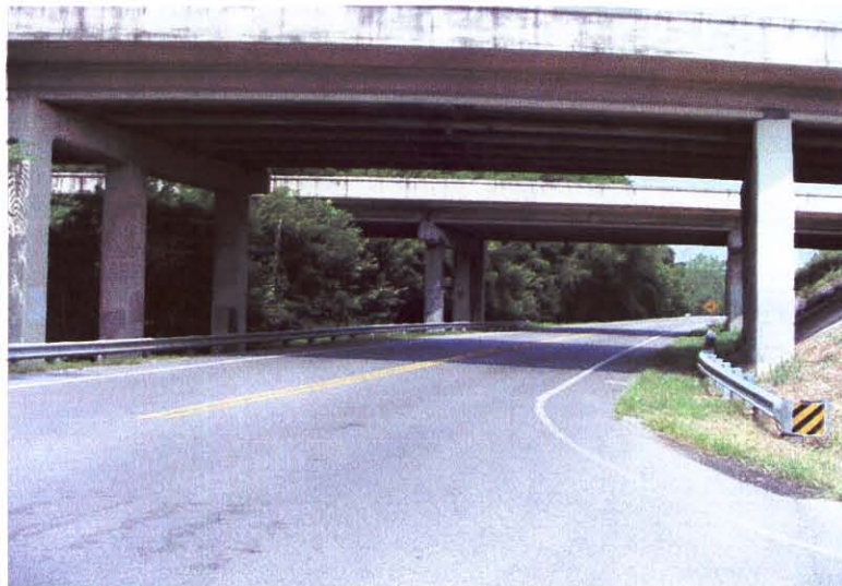
Looking Ahead on Route (94-106-5.88)
