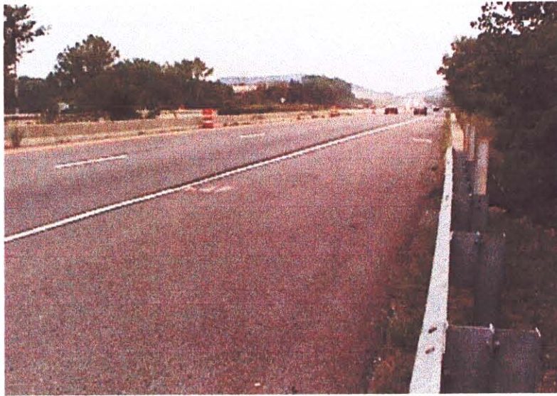
ACROSS TOP OF DECK
